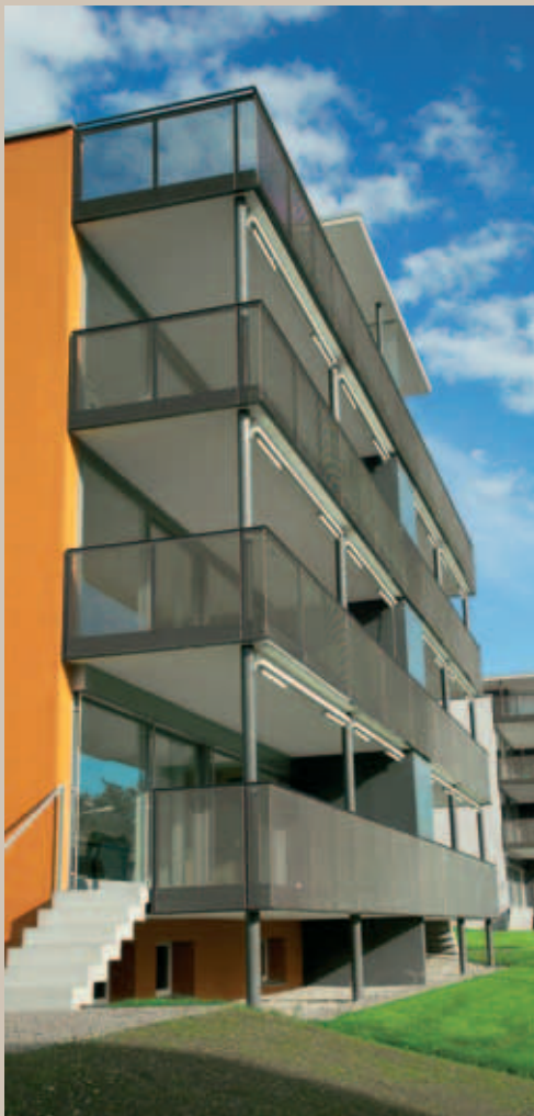
Project: Dachtler Partner AG (CH) - Mesh: Fils 5 - DL 62.5 x DC 20 (20) - av 7.5 x sp 1.5 mm Natural aluminium - Photo: Huber
