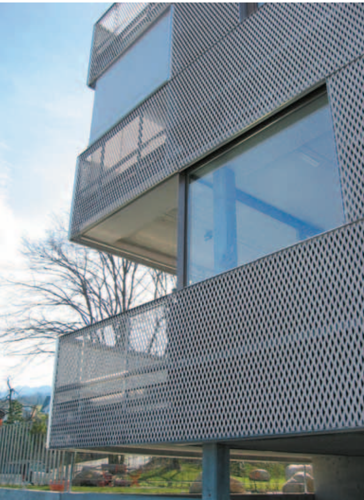
Project: Halter Generalunternehmung AG (CH) - Mesh: Ambasciata - DL 110 x DC 40 (52) - av 24 x sp 2 mm Peened aluminium - Photo: Metallpfister
