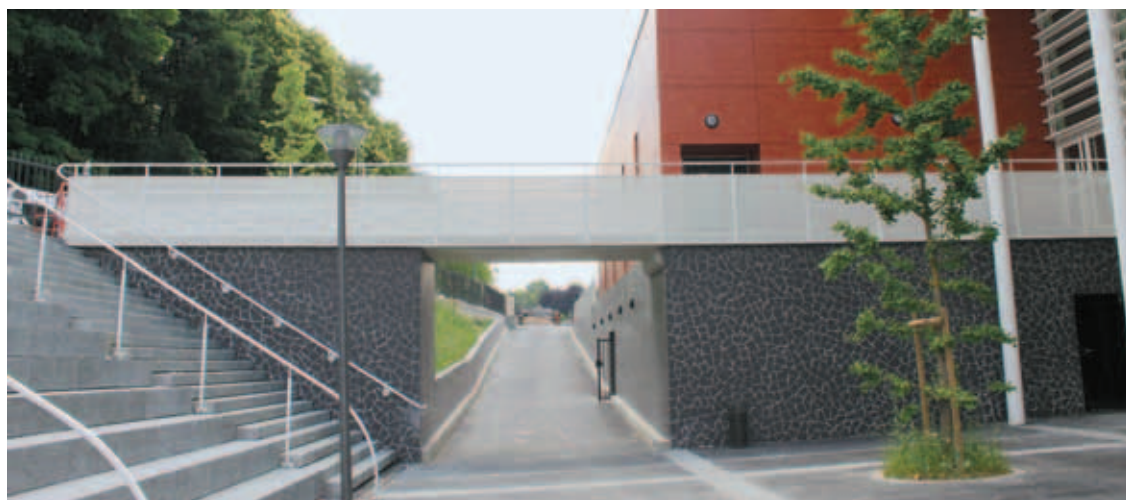
Project: Arch. M. Hesters (F) - Mesh: Academy - DL 115 x DC 40 (48) - av 20 x sp 1.5 mm Painted galvanised carbon steel
