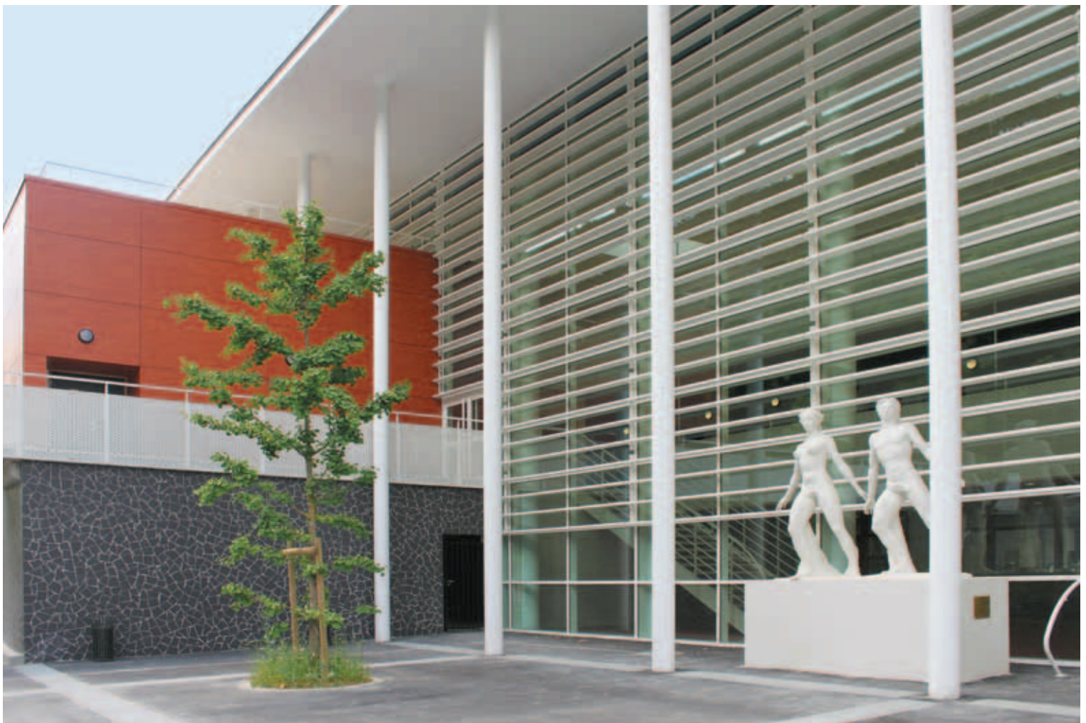
Project: Arch. M. Hesters (F) - Mesh: Academy - DL 115 x DC 40 (48) - av 20 x sp 1.5 mm Painted galvanised carbon steel
