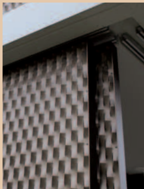
The sliding sunscreen installed as a part of a parapet can be positioned as required and guarantee visual comfort and optimum thermal performance.
