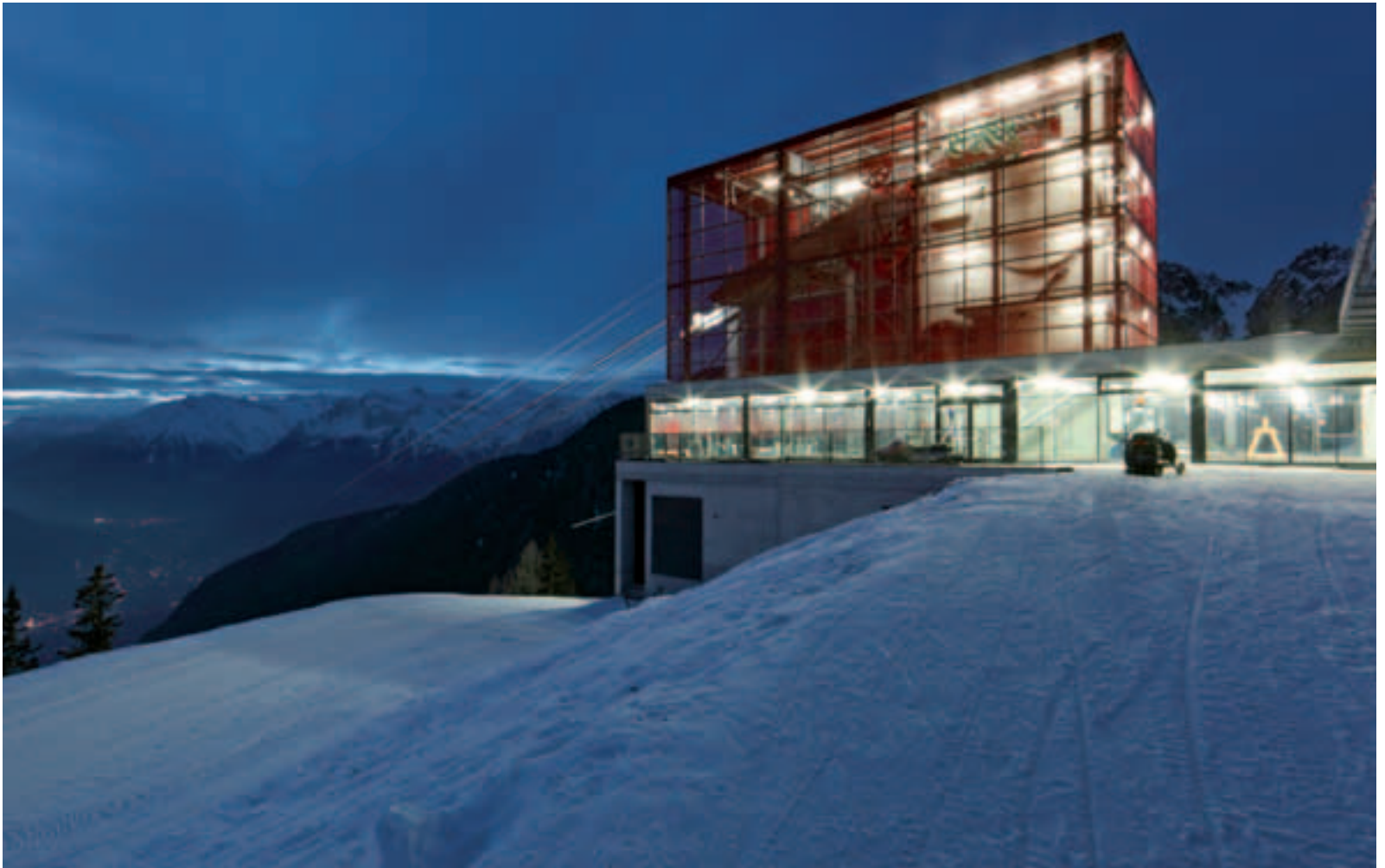
IVIGNA MERANO 2000 CABLE CAR STATIONS - BOLZANO (Italy) Design: Arch. Roland Baldi Photo: © Meran 2000 - Frieder Blicke
