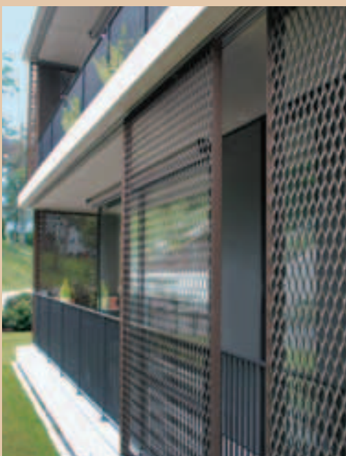
The sliding sunscreen installed as a part of a parapet can be positioned as required and guarantee visual comfort and optimum thermal performance.
