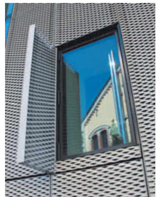
Vertical enclosure of the building, horizontal false ceiling, lateral “fins” as sunscreen for the windows to achieve the dual objective of facing and providing shade.
