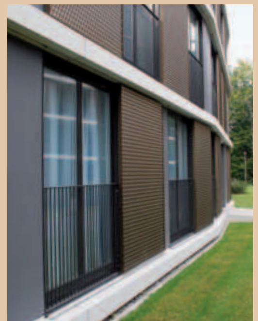
The sliding sunscreen installed as a part of a parapet can be positioned as required and guarantee visual comfort and optimum thermal performance.
